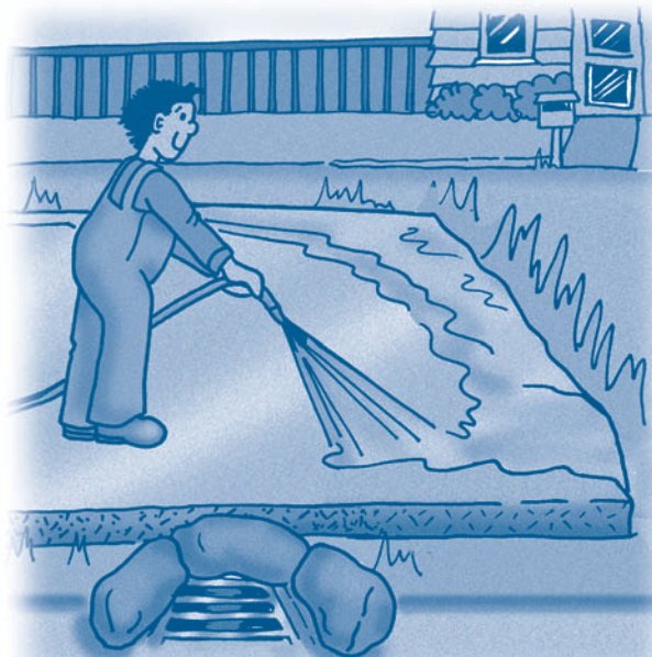
Make sure drains are protected from wash down run-off.
